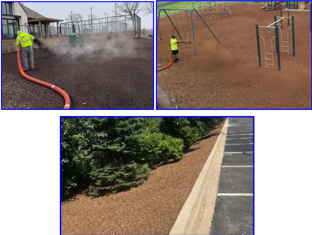
Mechanical blown-in application finished result
